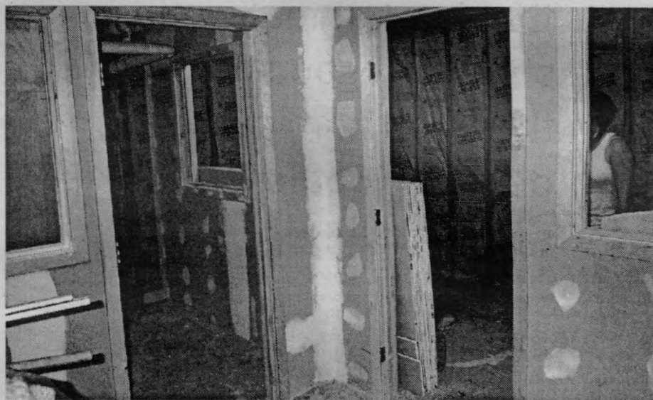
The new digs: the WXBC renovation is already underway
