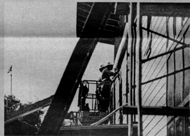
Construction Workers: doing their job on Campus Road Dorms.
