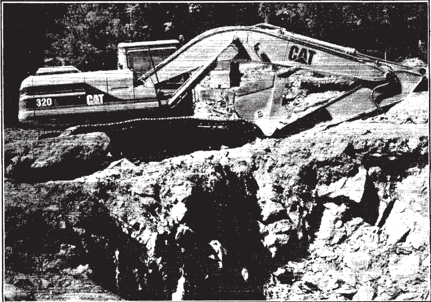
Construction equipment outside the F.W. Olin Humanities Building as ground is broken for the Language Center.
