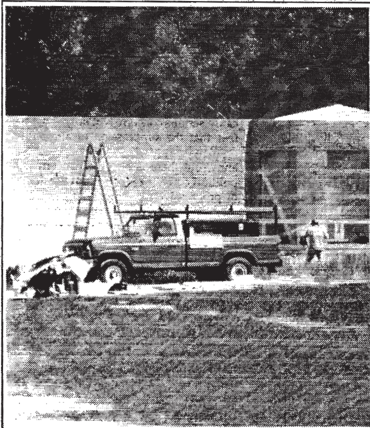
The partially-completed Black Center.
