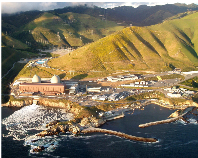
The entirety of Diablo Canyon's facility from the air. (Figueroa 2005).
