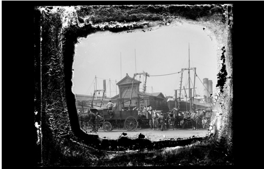
Figure 2.1. Waterfront traffic at Pier 46 (Troy Line), New York City. Undated. New York Historical Society. New York, NY.
