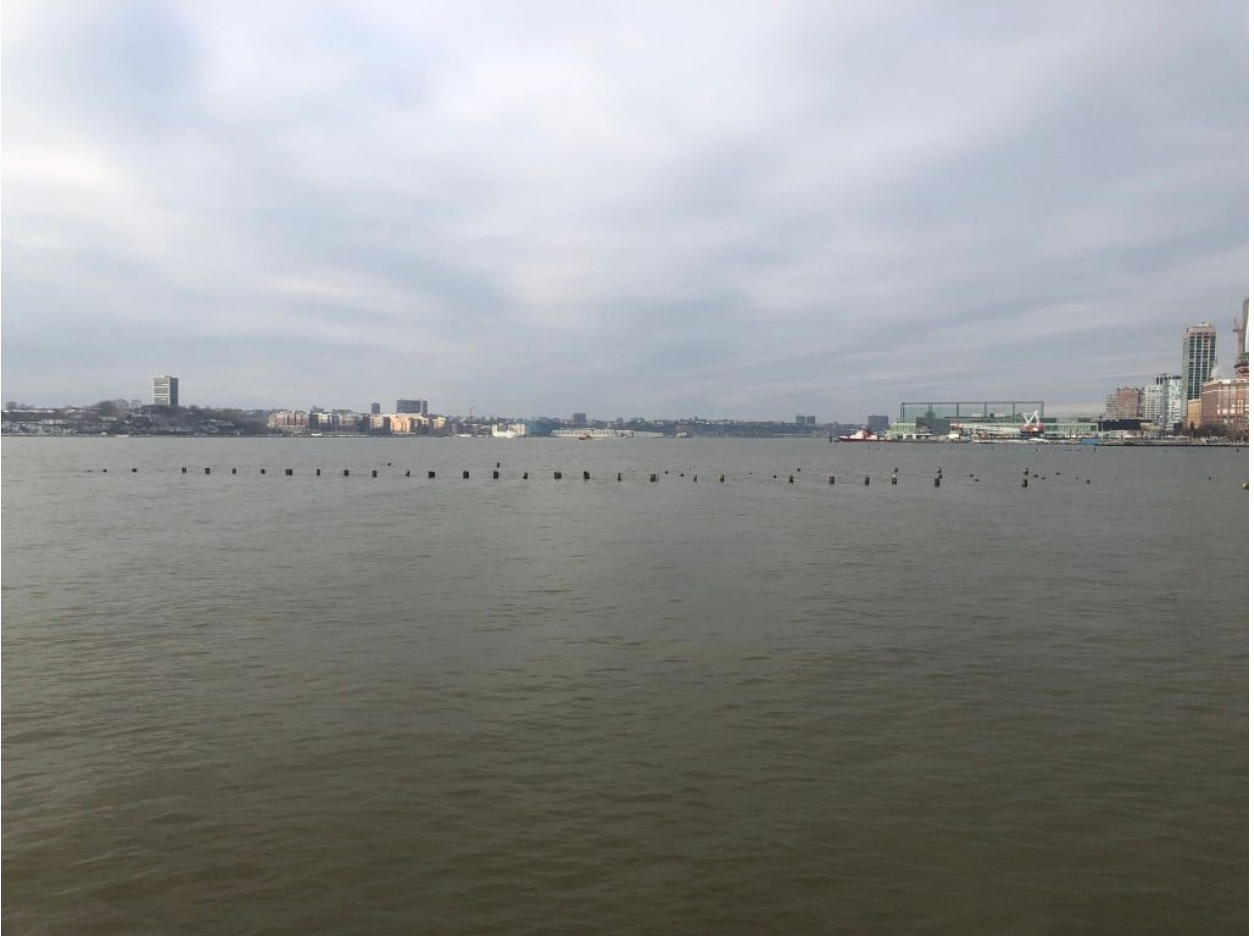
Figure 2.32. The original pilings of a pier. 2019. New York, NY.
