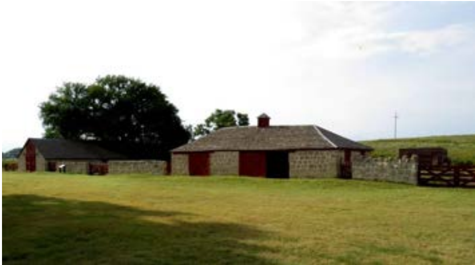
Shearing and lamb building at far left, shop and stable in center 60
