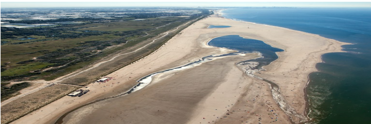
above) Image #2 of a Sand Motor in the Netherlands.
