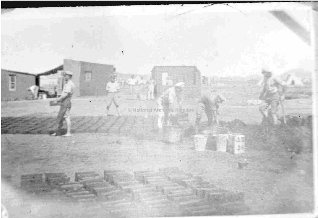
Figure 4: NAN: Aus camp, Germans making bricks to build housing
