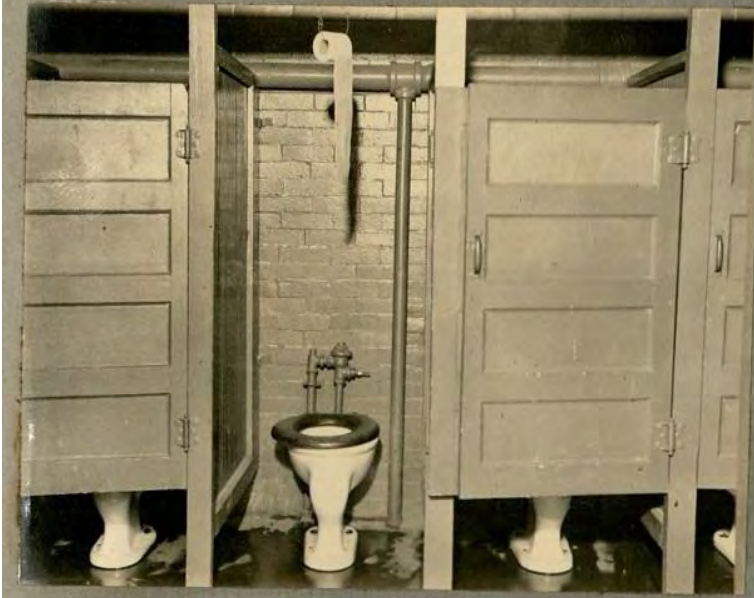
Figure 2.18: Department of Parks NYC, Red Hook Park Comfort Station, Comfort Stations Survey of 1934 .
