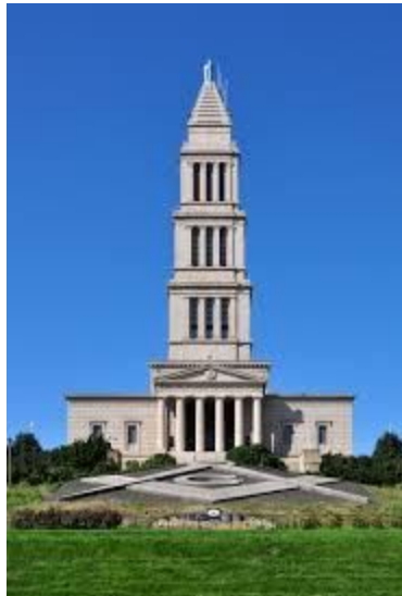
Front view of George Washington Masonic National Memorial. Unknown photographer and date.
