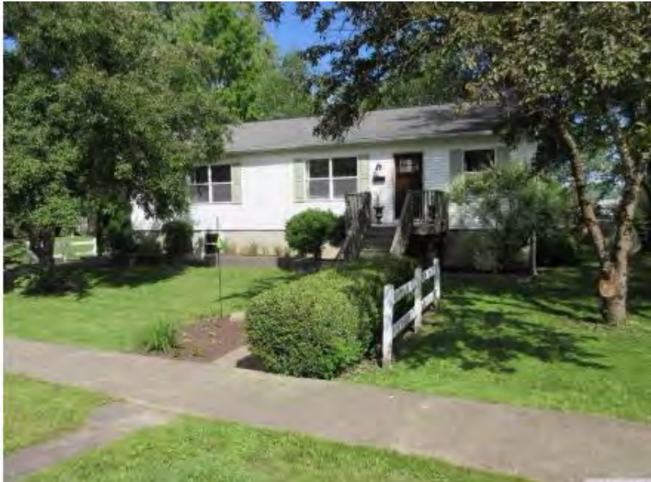
Figure 1 : Photo of the front yard from zillow.com listing, early Summer 2017.
