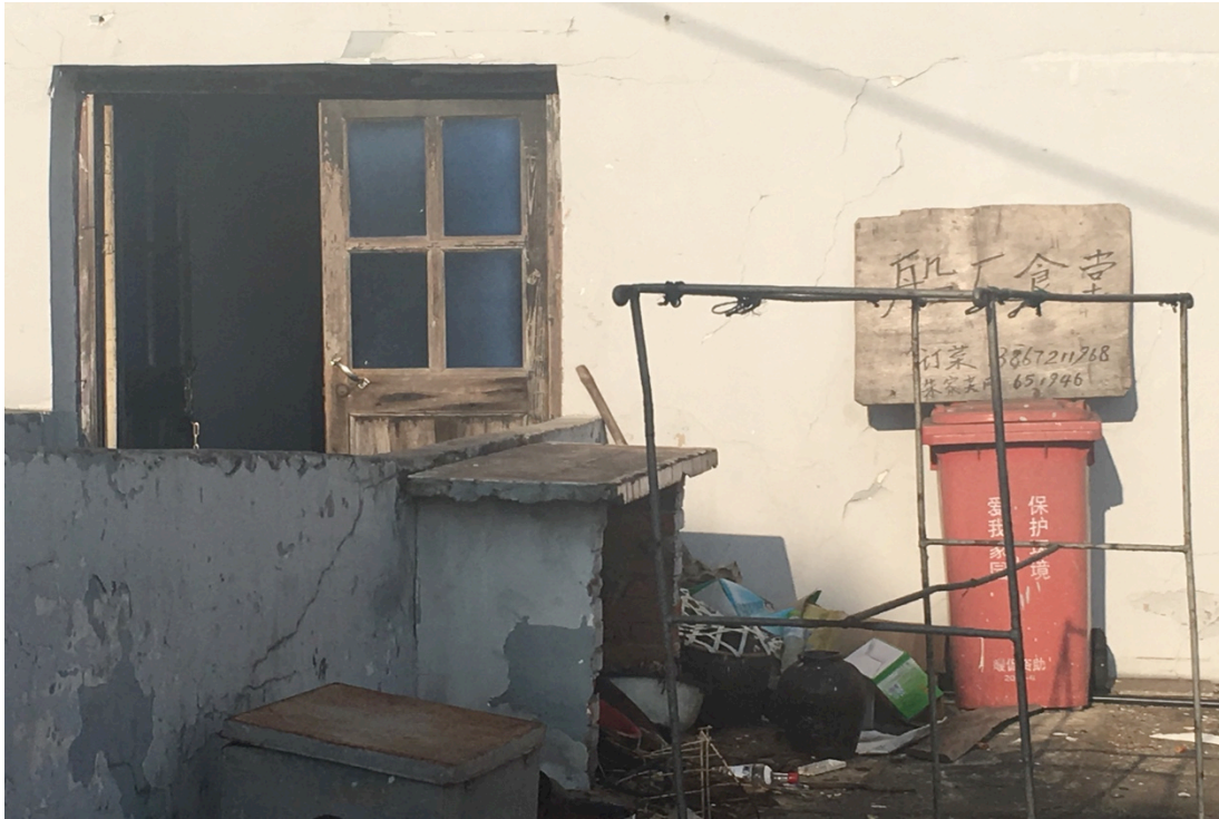
Old houses, half pulled down. This house had previously been used as a cafeteria for fish workers.
