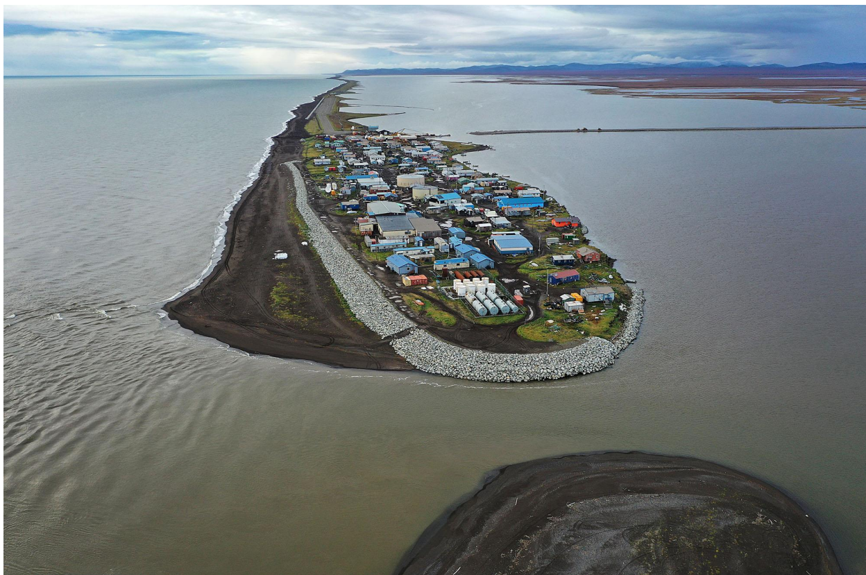
Figure 3. The Native Village of Kivalina, seen from above. Boulders have been shipped in and positioned to construct a sea wall to protect the village against storm surges. ( The Atlantic )
