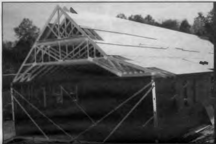
Building version: Construction has begun on the new Freshman Octuples.
