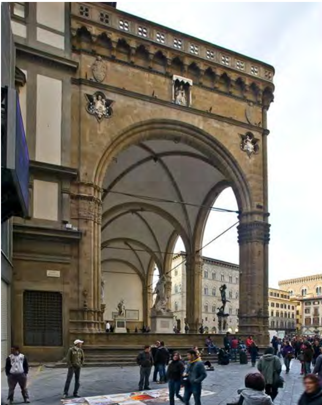
Figure 14a. Alternate view, On the side of Loggia, between the early Renaissance structure and the Palazzo Vecchio. The interior vaulted ceilings as well as the openness of the loggia are shown. (photograph by Ralph Lieberman, 2009)
