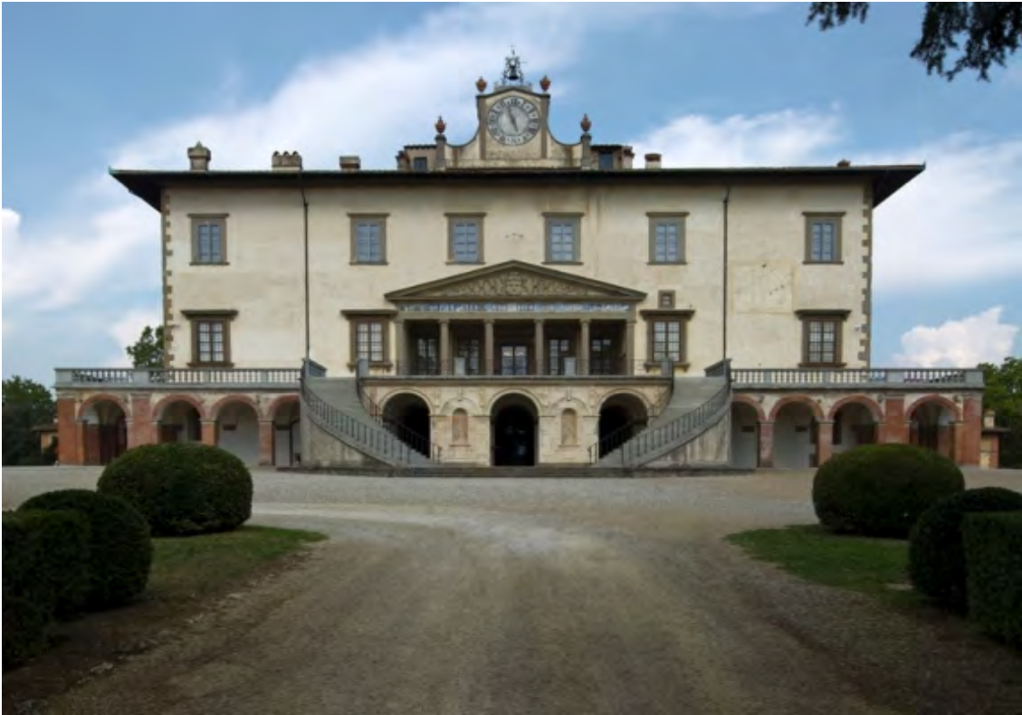
Figure 36. Front façade and approach to Poggio a Caiano by da Sangallo c. 1485 for Lorenzo de' Medici (Museums of Florence website)
