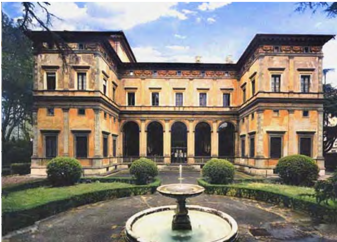
Figure 9. Back façade of Villa Chigi (later the Villa Farnesina) for Agostino Chigi, c. 1510, Rome; facing north, with loggia garden loggia at center (Academic Nazionale di Lincei; lincei.it)
