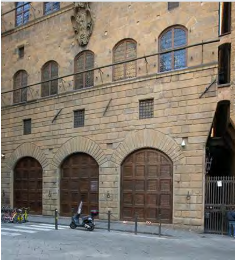
Figure 15. Davizzi detail of front; the loggia doors, three arcuated bays; in quattrocento Florence, the wooden doors were not a part of the structure. The Davanzati crest had not arrived to the façade either. (photograph by Ralph Lieberman 2009)
