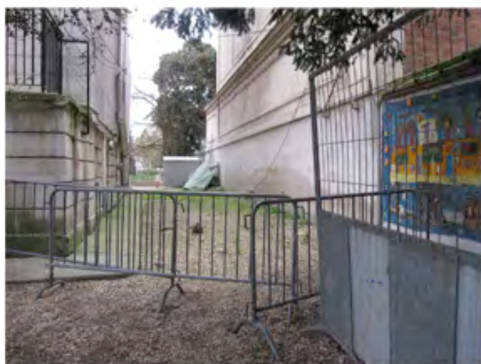
Fig. 73 Passage to the side of the Haussman building
