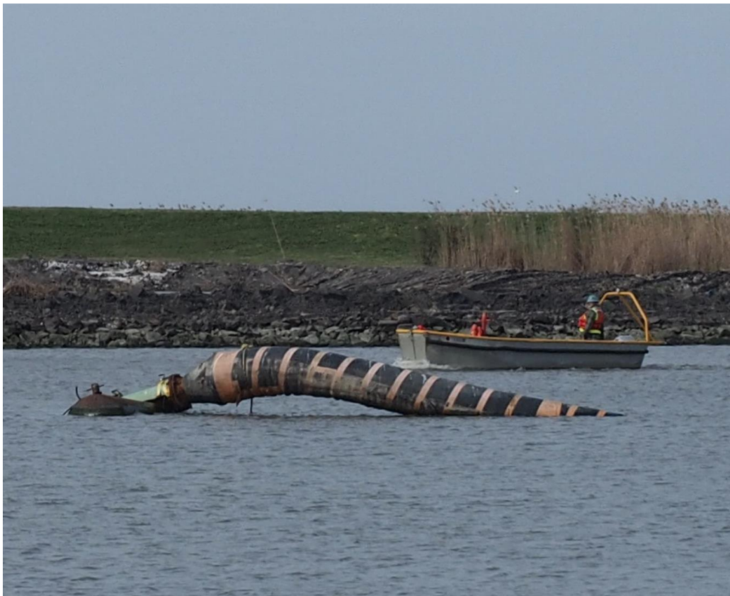
16. USACE pipeline dredging project at a harbor in Plaquemines Parish.
