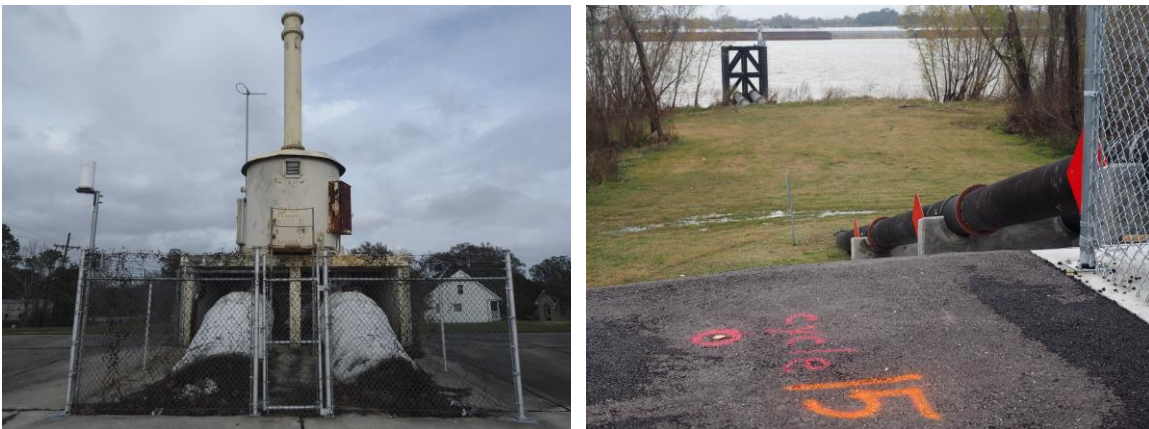
Fig. 4. Pumping stations along the levee at Sauv 's Crevasse (personal photos).
