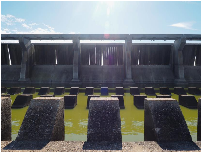
Fig. 5. BCS viewed from the floodway – retention basin and needles (personal photo).
