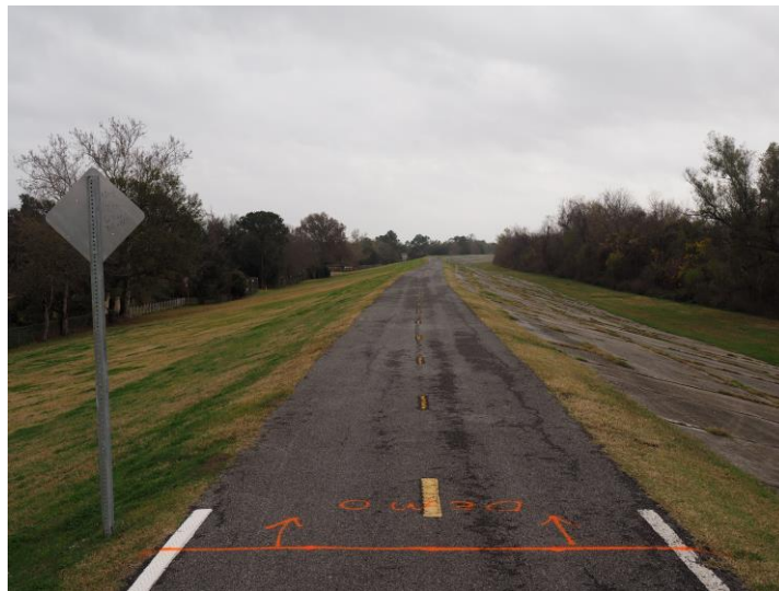
Fig. 3. The levee at Sauv e's Crevasse (personal photo).
