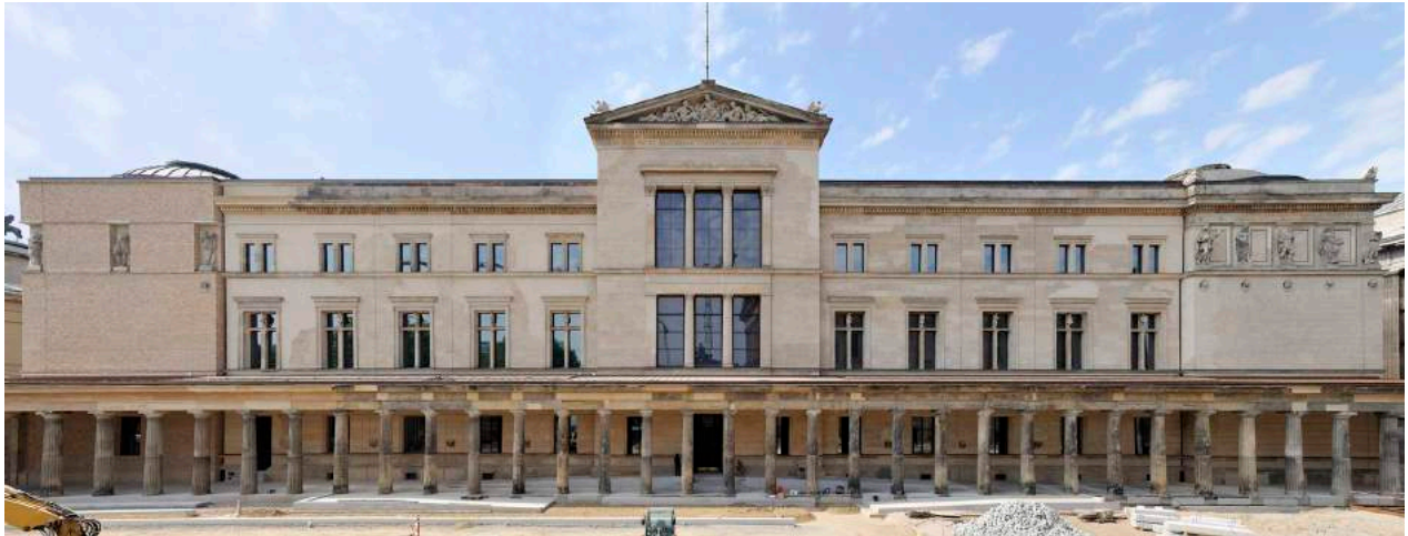
Figure 2.2. The west façade and entrance to the Neues Museum, c. 2009.
