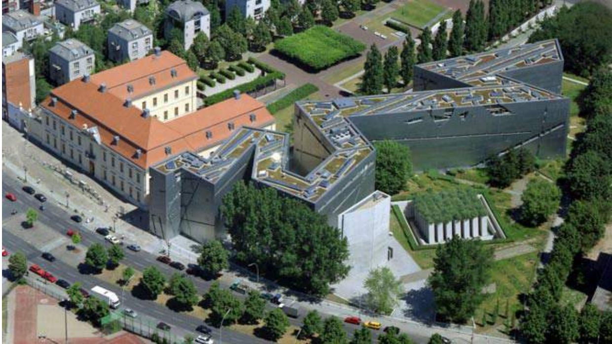
Figure 3.2. The Jewish Museum, Berlin and its surrounding buildings. Source: Bird's eye view of Jewish Museum, Open Buildings, digital photograph, Berlin, http://openbuildings.com/buildings/jewish-museum-berlin-profile-9719 .
